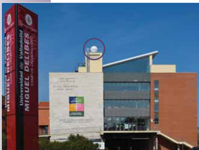
▲ Dartcom X-Band EOS System at the University of Valladolid, Spain, with the antenna system (circled) installed on top of a lift shaft
